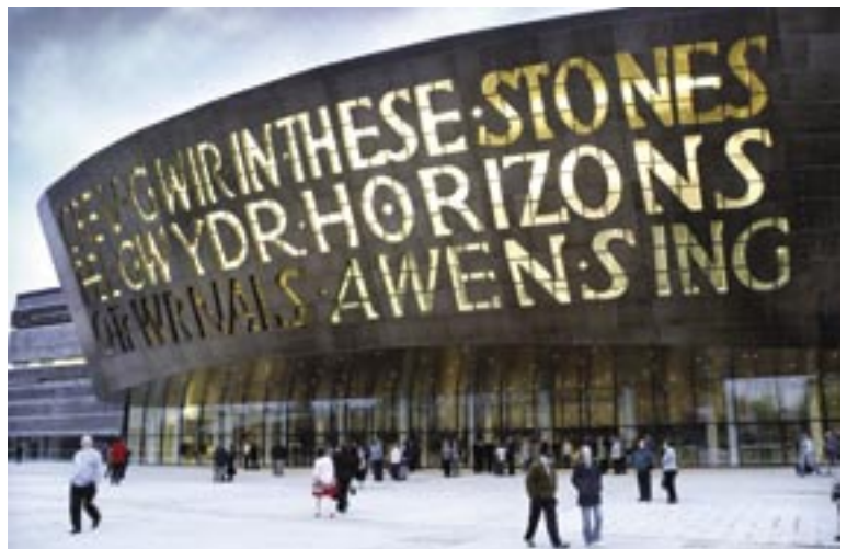
Project: Wales Millenium Centre Contractor: GHT Plastering Services
